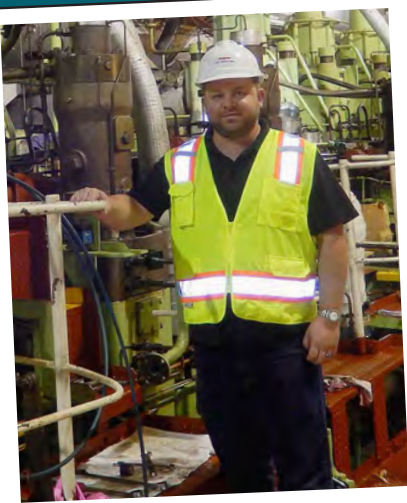
Port Engineer Keith Deirup by the main engine heads onboard the APL KOREA.
