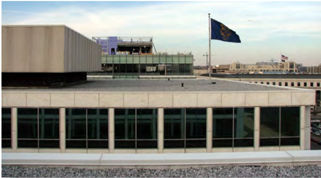
The north tower of 444 North Capitol Street (taken from the south tower) before construction.
