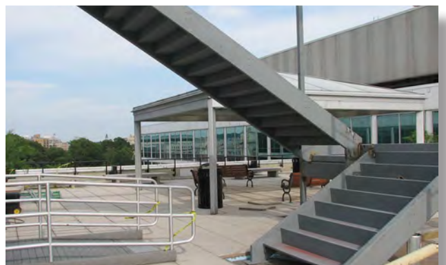
The two halves of the steel staircase is fitted together.
